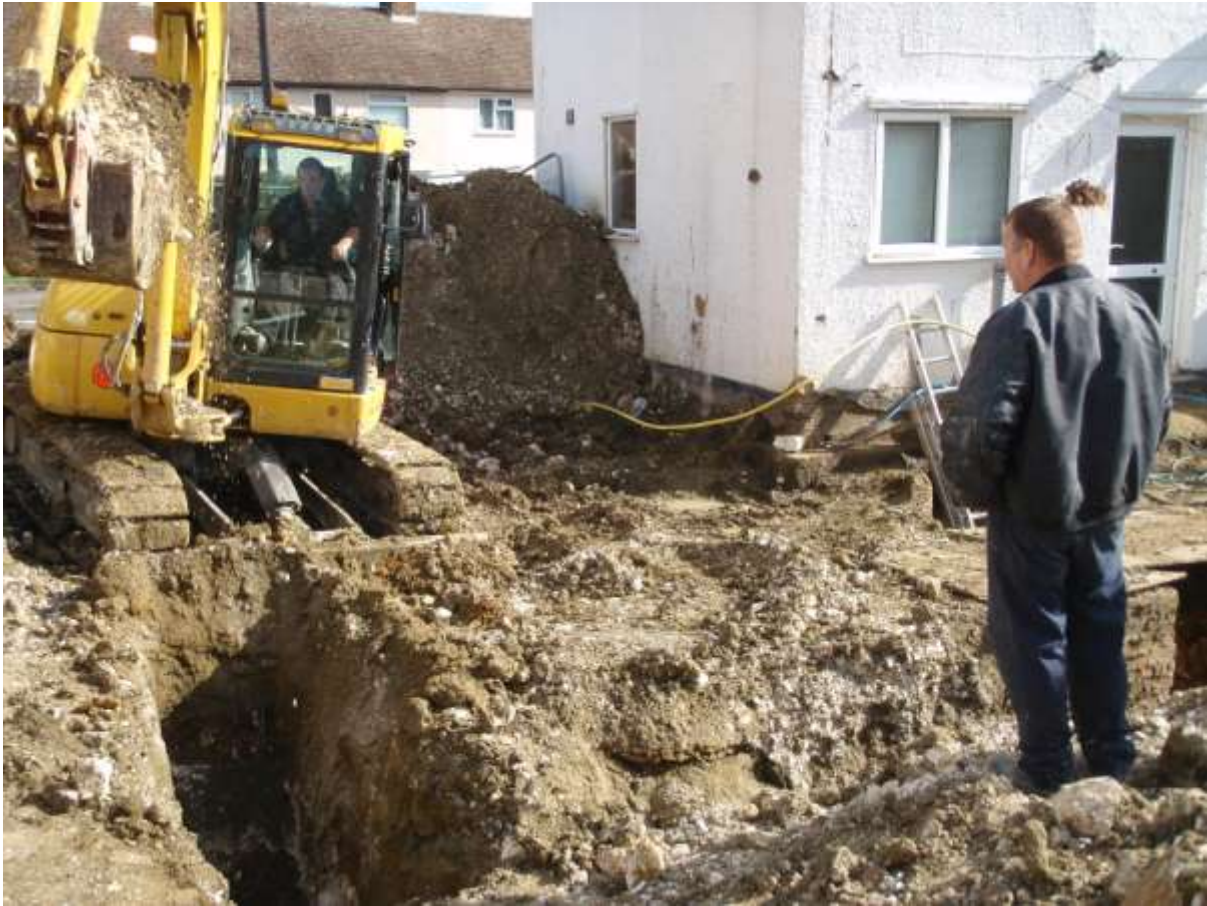
Plate 4. Foundation trench showing geology (facing north)
