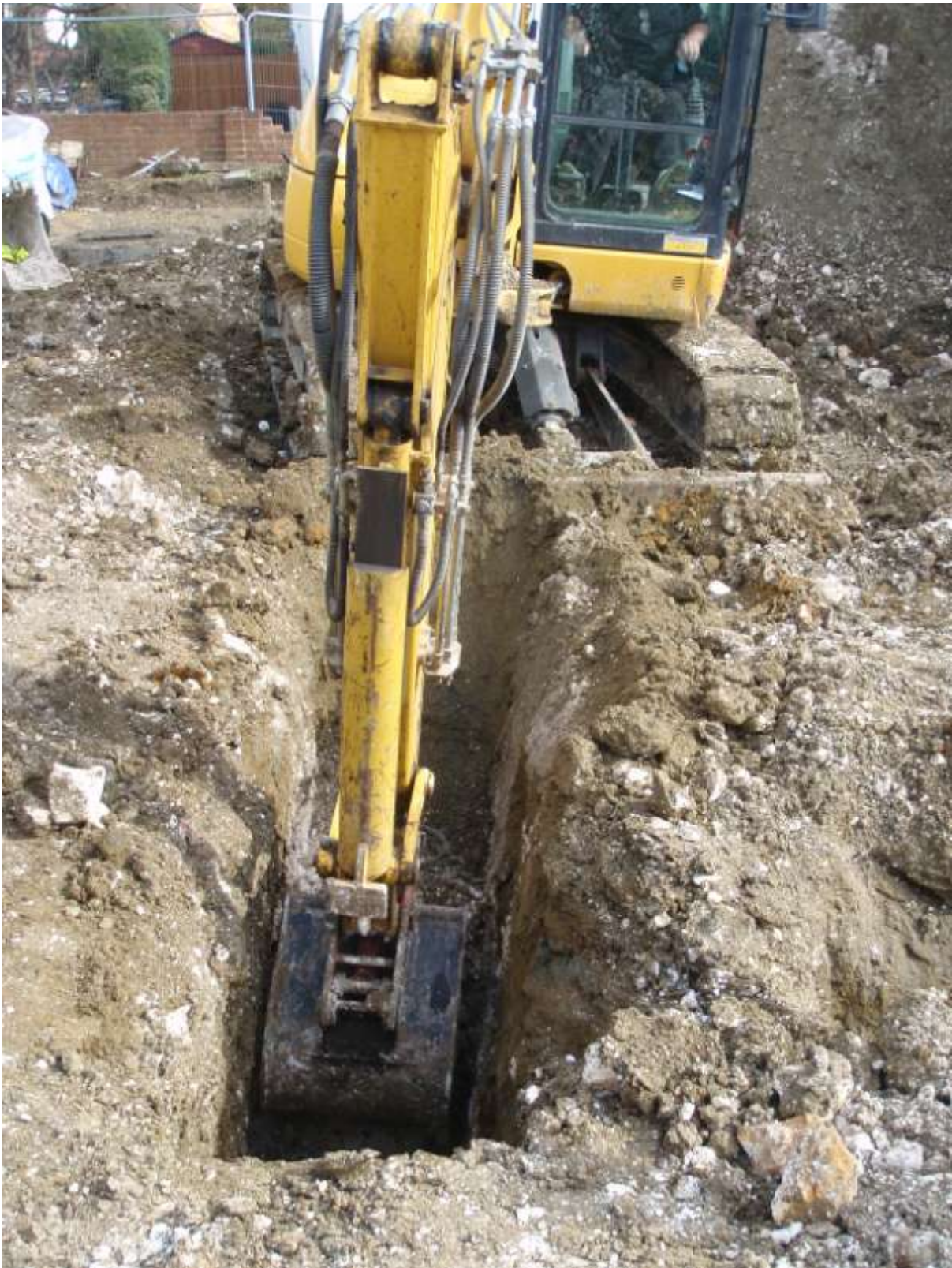
Plate 2. General view of site with foundation trenches excavated, (looking north)
