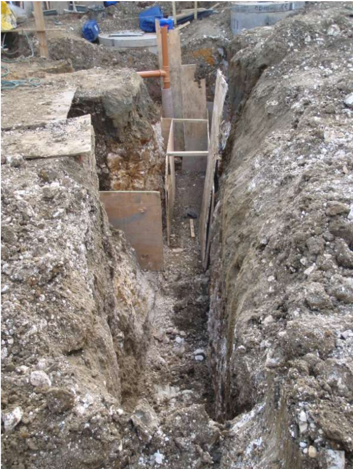
Plate 3. The site showing ground works for drain connection (looking east)
